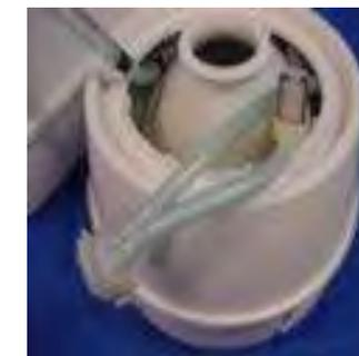
Remove the flush tube including electric valve.
